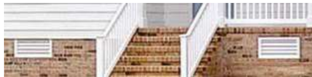
Example Foundation Vents
