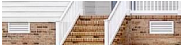
Example Foundation Vents
